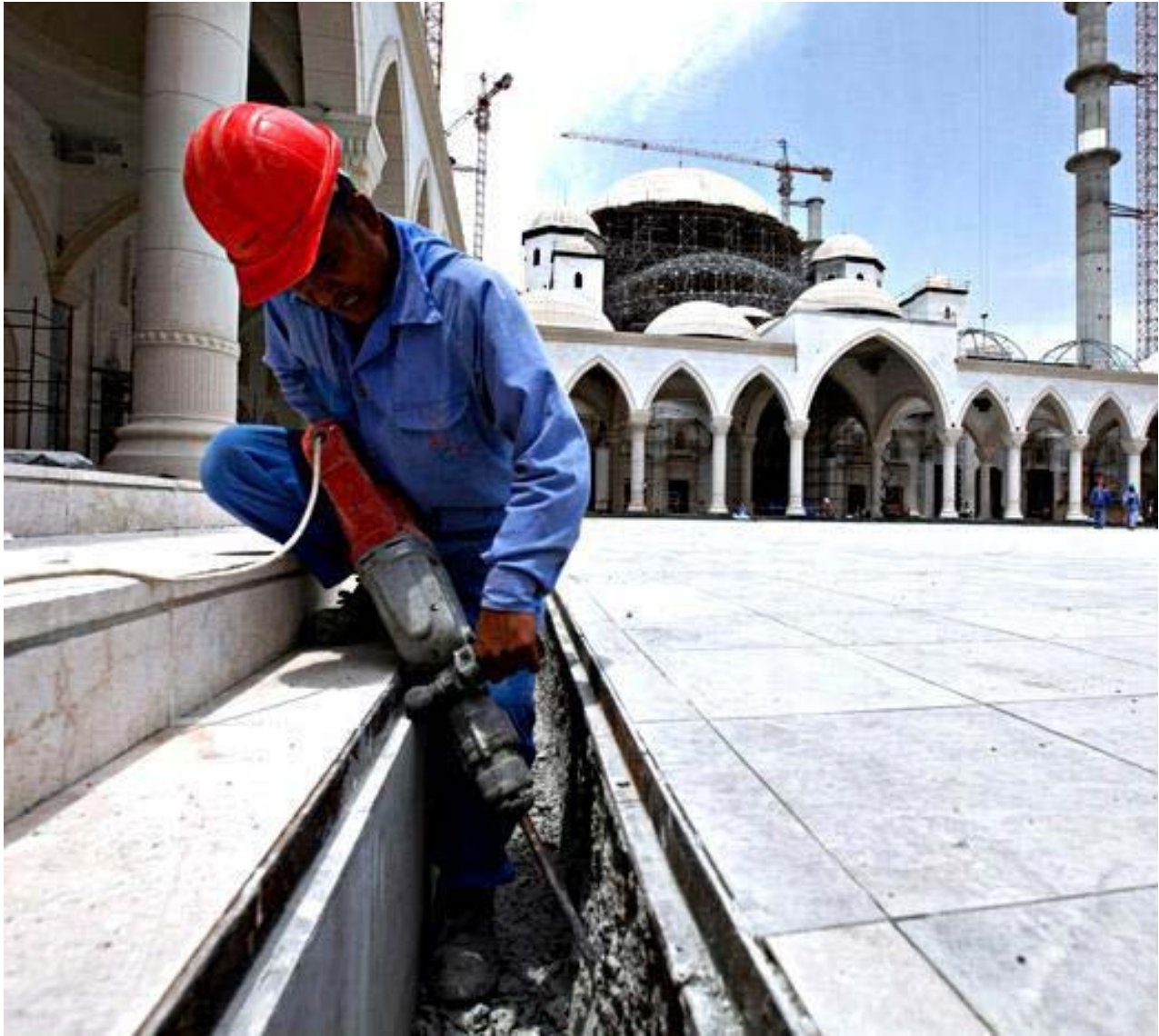
FUJARIAH, UNITED ARAB EMIRATES - July 31, 2012 - Siddiki Sarkar chisels away some of the cement wall that will be covered with plastered in this drainage trough along one side of the mall of the Sheikh Zayed Mosque mosque being built in Fujariah City, Fujariah, July 31, 2012. (Photo by Jeff Topping/The National)
